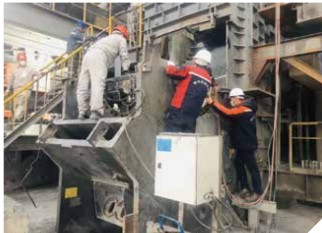
Jaw Crusher Maintenance
