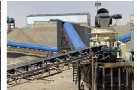
Inner Mongolia Iron Ore Project, Capacity: 300 tons per hour
