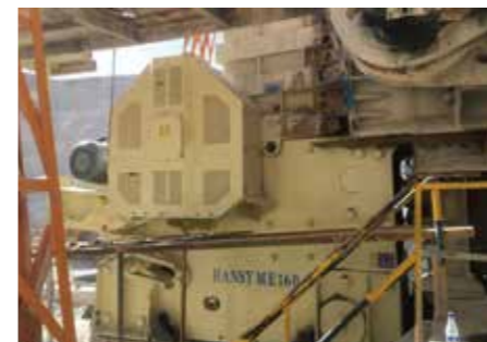
Inner Mongolia Molybdenum Ore Project, Capacity: 800 tons per hour
